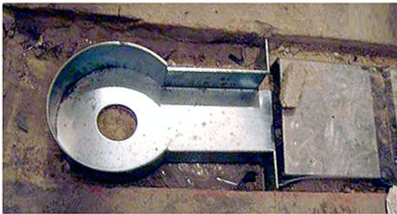
Figure 71 Cable Conduit For On-Grade Floor Anchor Kit
