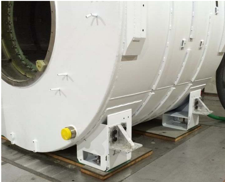
Figure 6-14 Magnet installed on surface mounted vibroacoustic damping mats*
