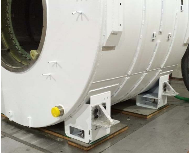
Figure 7-12 Magnet installed on surface mounted vibroacoustic damping mats*
