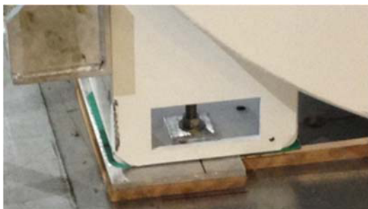
Figure 6-13 Magnet lowered on vibroacoustic mat
